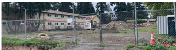
Cedar Tree Apartments, 643 NE 162nd Ave. Land clearing underway
