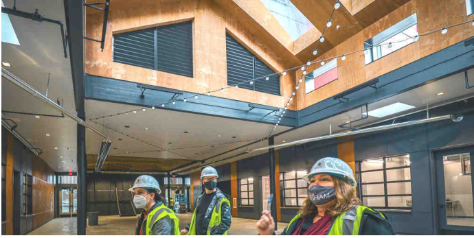
Construction progress, Rockwood Market Hall. Photo: City of Gresham
