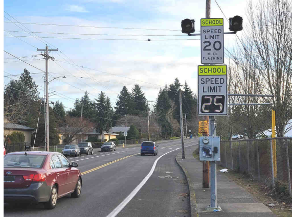
Radar speed sign at NE 172nd Avenue & NE Clackamas Street
