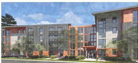
Albertina Kerr Workforce and Inclusive Housing. East entrance, Gresham campus. Architects Image
